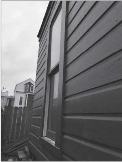
10. SIDING DETAIL TO BE REPLACED WITH MATCHING
