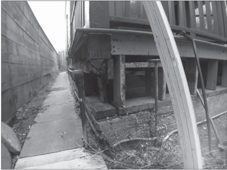
11. NORTHWEST CORNER SHOWING CRUMBLING FOUNDATION AND ROTTEN FRAMING, TYPICAL THROUGHOUT
