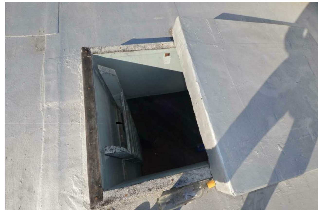
EXISTING ROOF HATCH ACCESS LADDER FROM DECK BELOW
