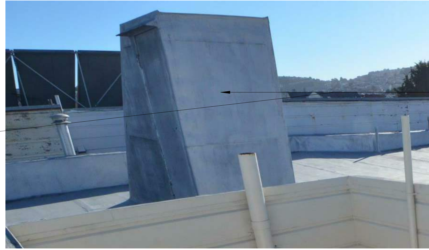
EXISTING ROOF PENTHOUSE
