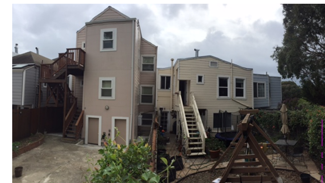
3 EXISTING REAR (NORTH) COMPOSITE PHOTO 1/4" / FT.
