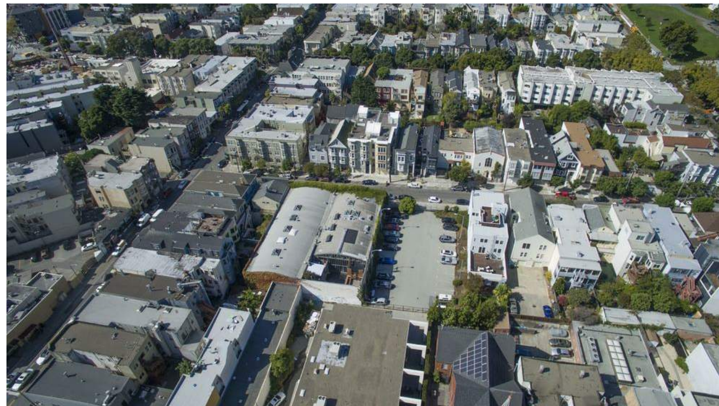
AERIAL VIEW - SUBJECT LOT (LOOKING WEST)
