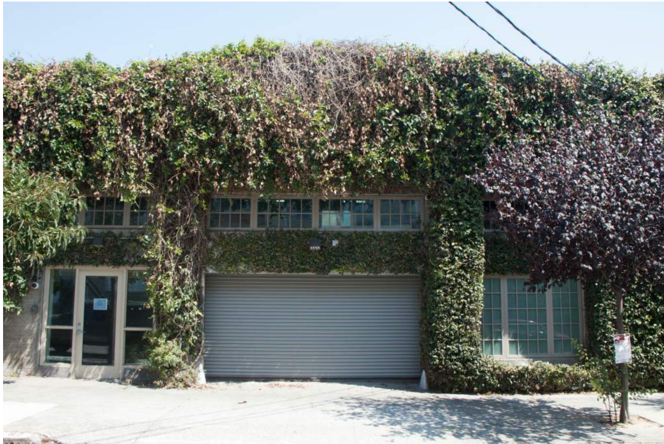
67 BELCHER WEST FACADE
