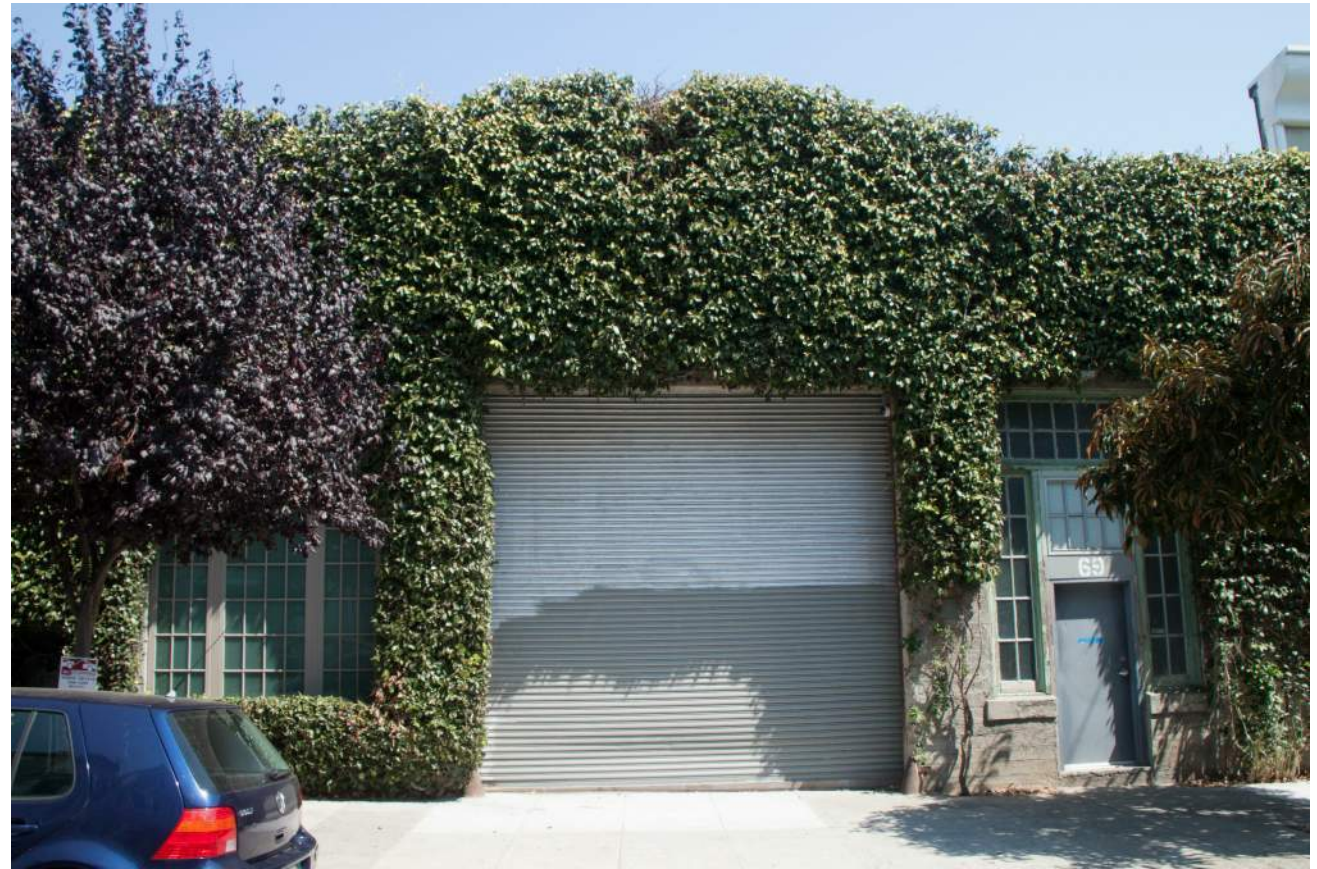
69 BELCHER WEST FACADE
