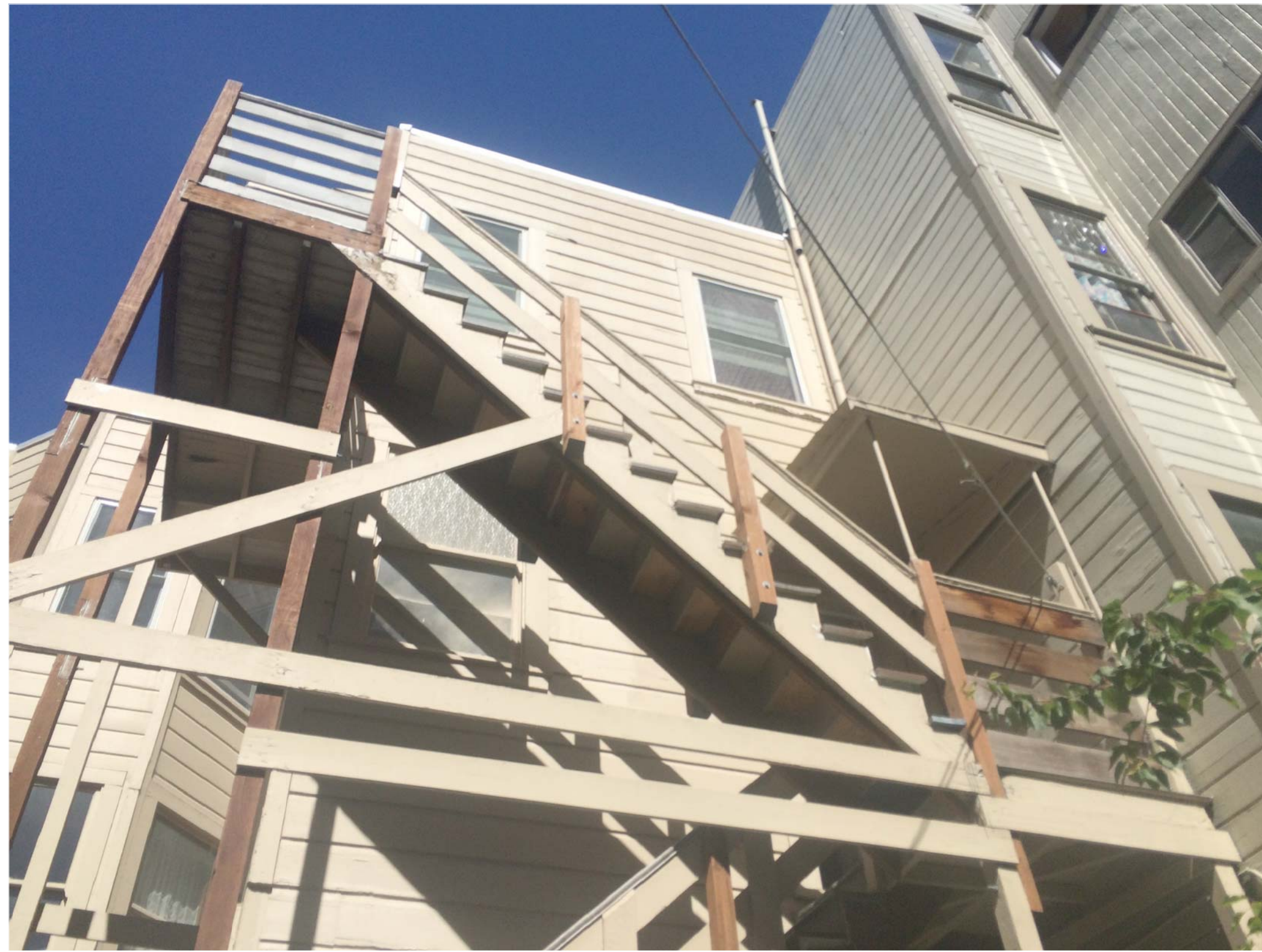
EXISTING REAR VIEW OF SUBJECT PROPERTY
