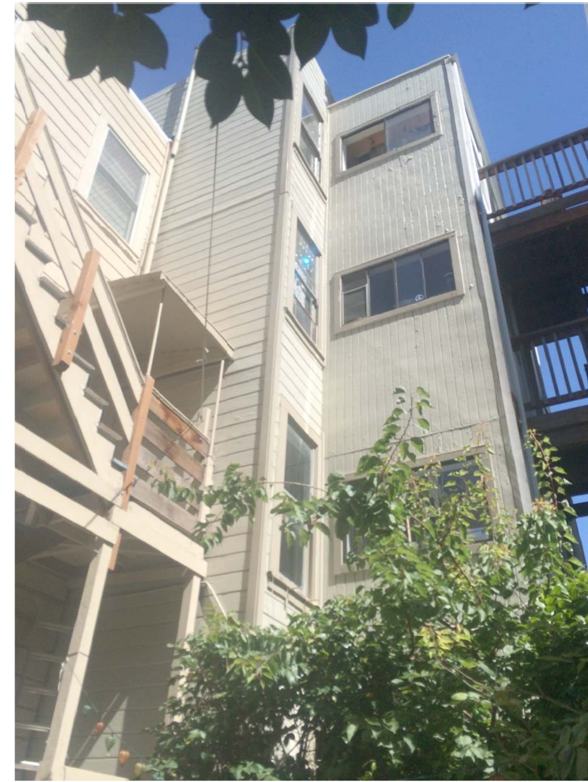
EXISTING REAR VIEW OF ADJACENT BUILDING ON THE NORTH
