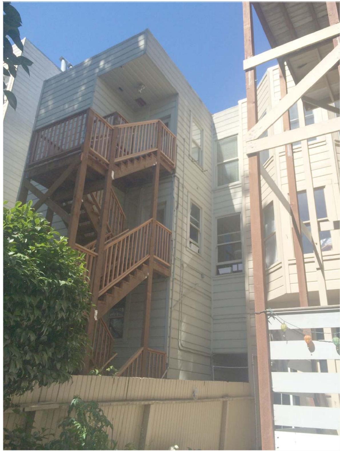
EXISTING REAR VIEW OF ADJACENT BUILDING ON THE SOUTH
