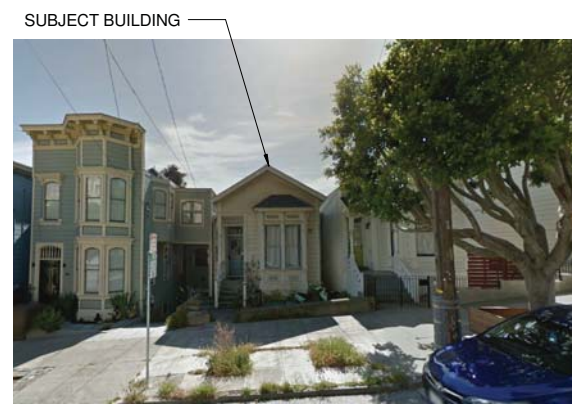
6 FRONT FACADE OF THE SUBJECT BUILDING 3/64" = 1'-0"
