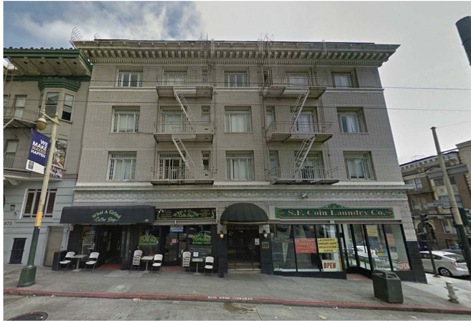
1. BUILDING STREET VIEW (POST ST)
