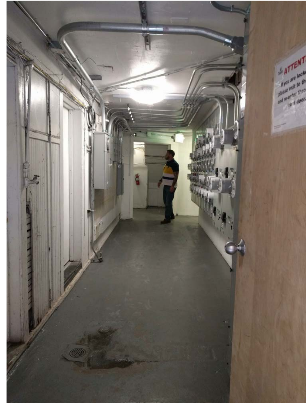
6. BASEMENT INTERIOR HALLWAY
