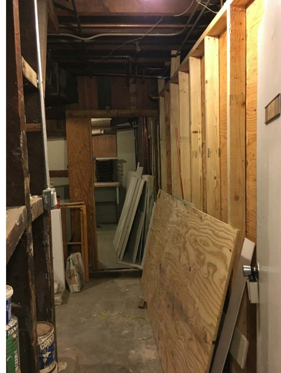
7. EXISTING STORAGE SPACE
