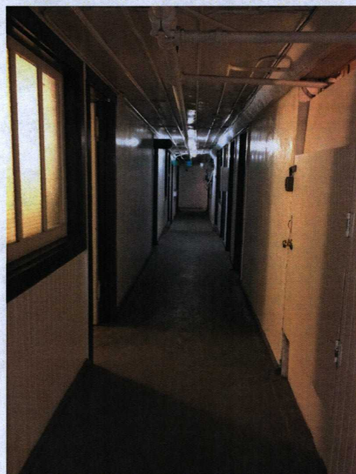
5. (E) BASEMENT CORRIDOR
