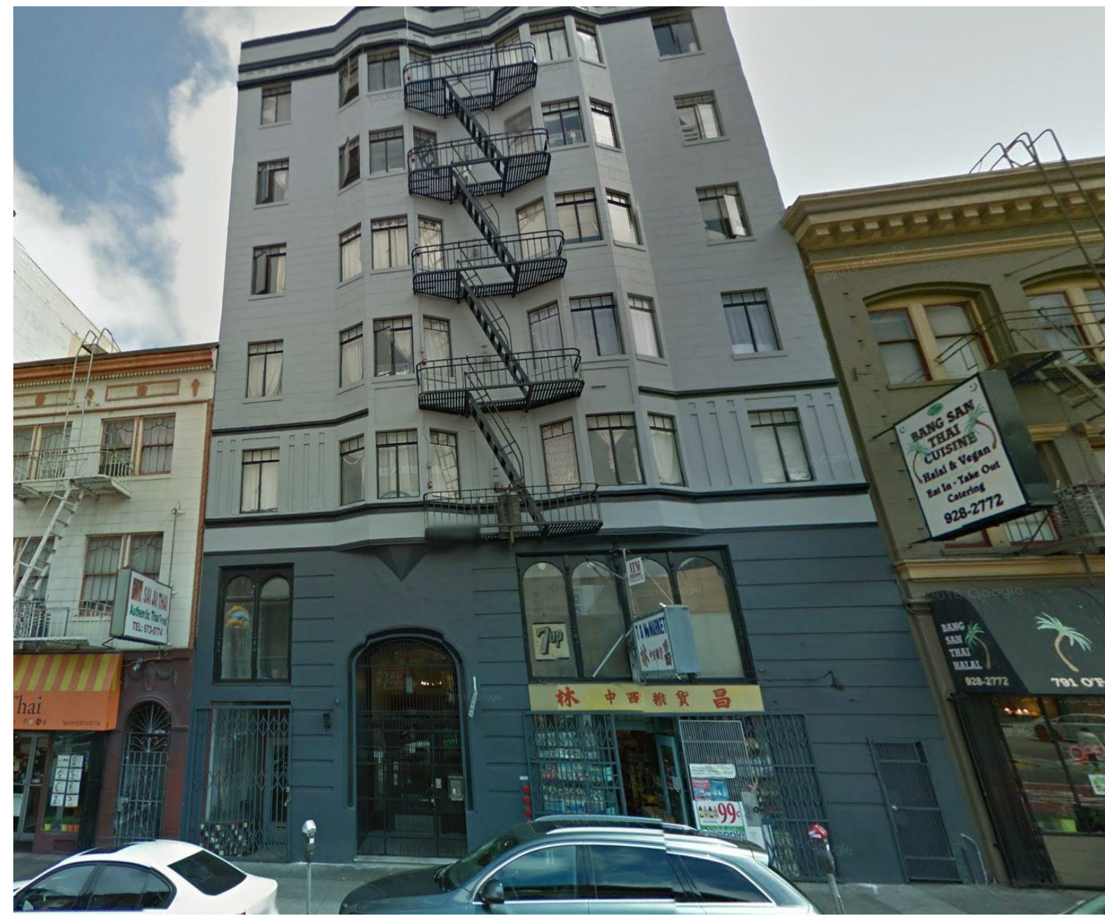
1. EXISTING FRONT FACADE OF THE SUBJECT BUILDING
