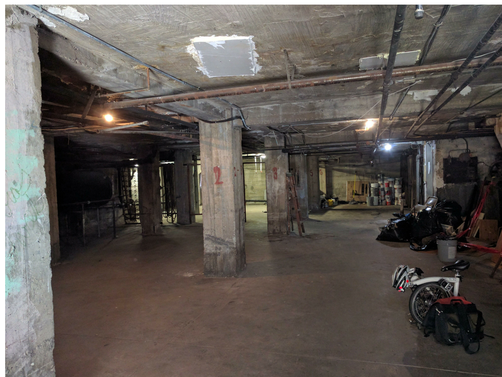
5. BASEMENT STORAGE ROOM
