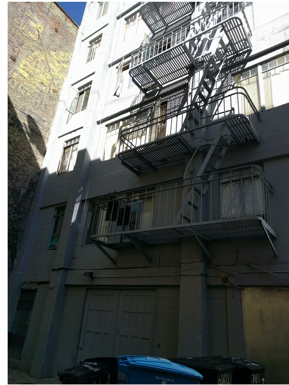
2. BUILDING REAR VIEW
