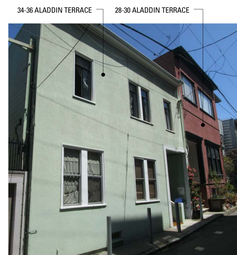
4 Existing Photos - north 3
