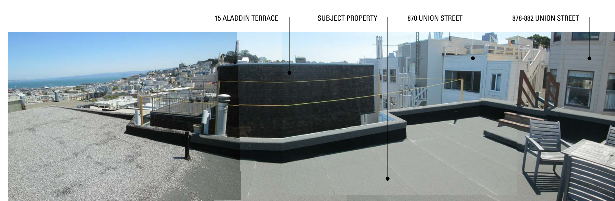
12 VIEWS FROM SUBJECT PROPERTY ROOF
