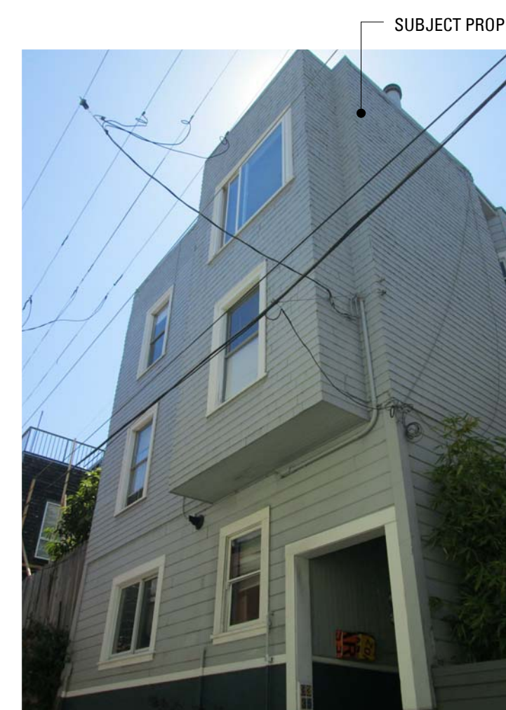
3 FRONT OF SUBJECT BUILDING
