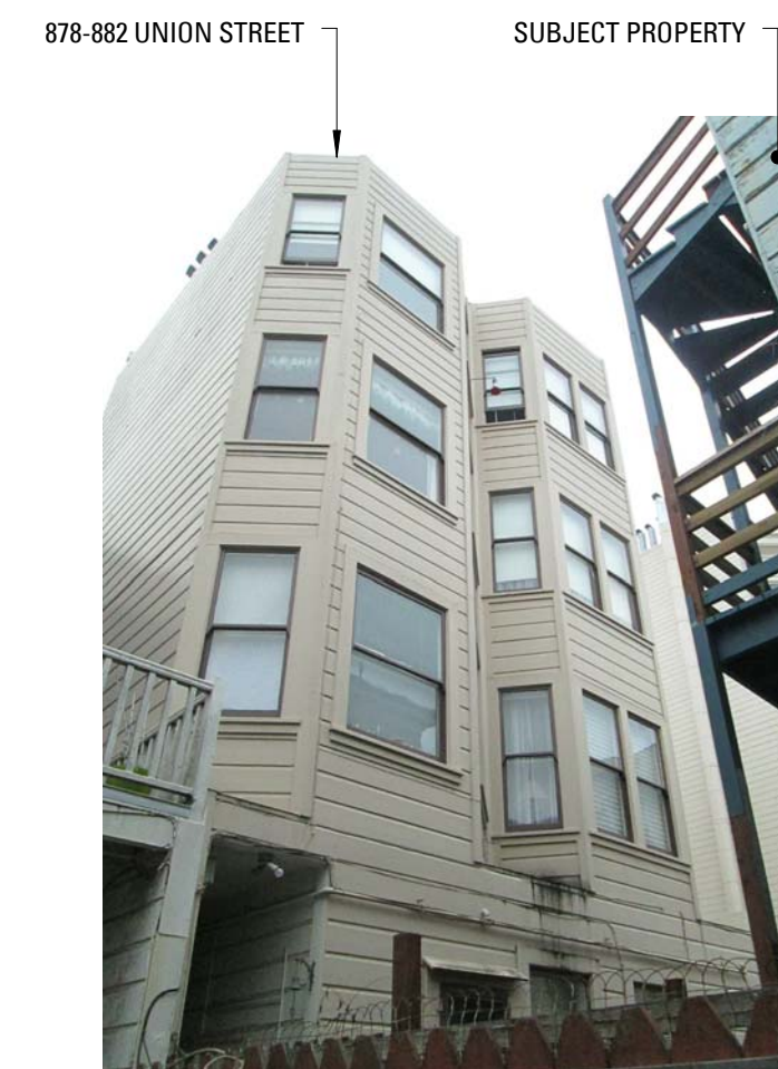
8 ADJACENT BUILDING TO SOUTH
