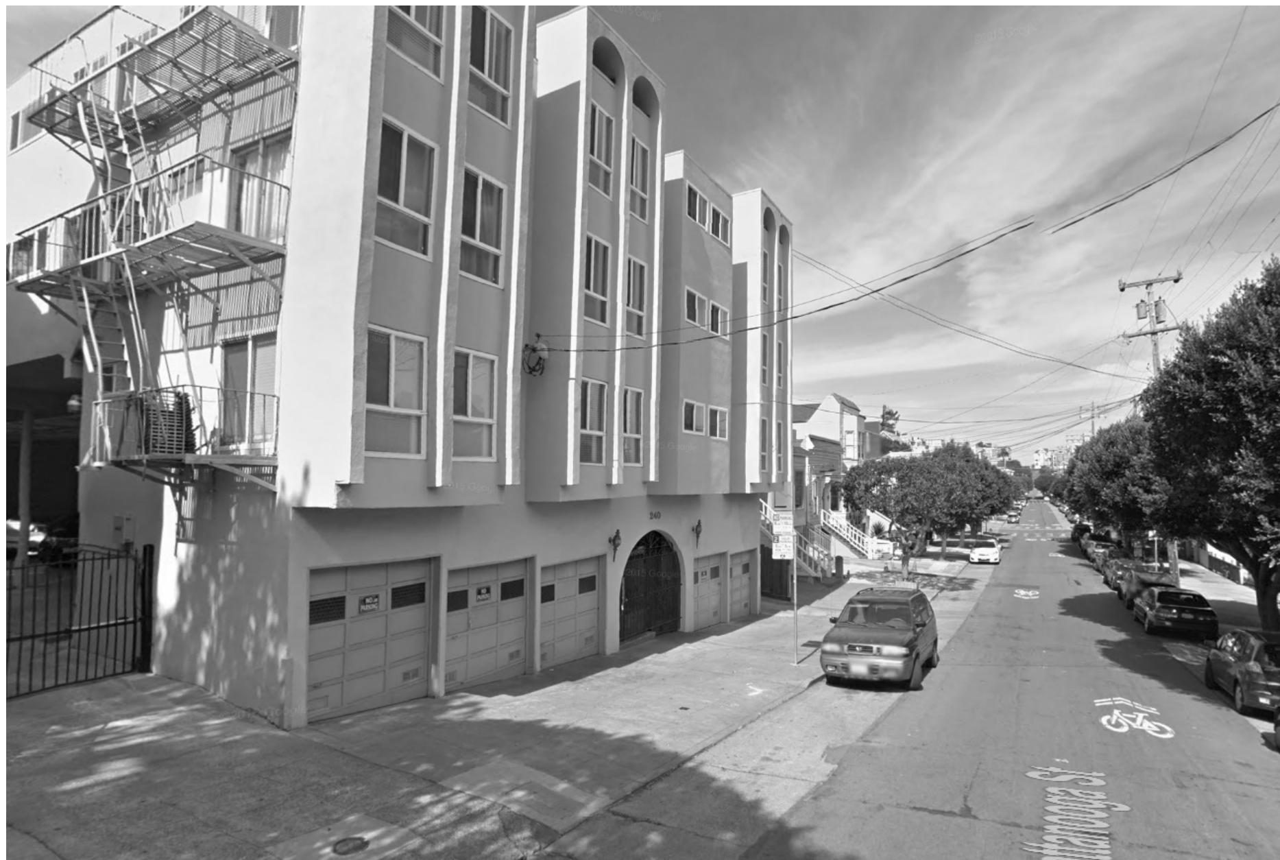
NEIGHBORS VIEW: FACING NORTH WEST
