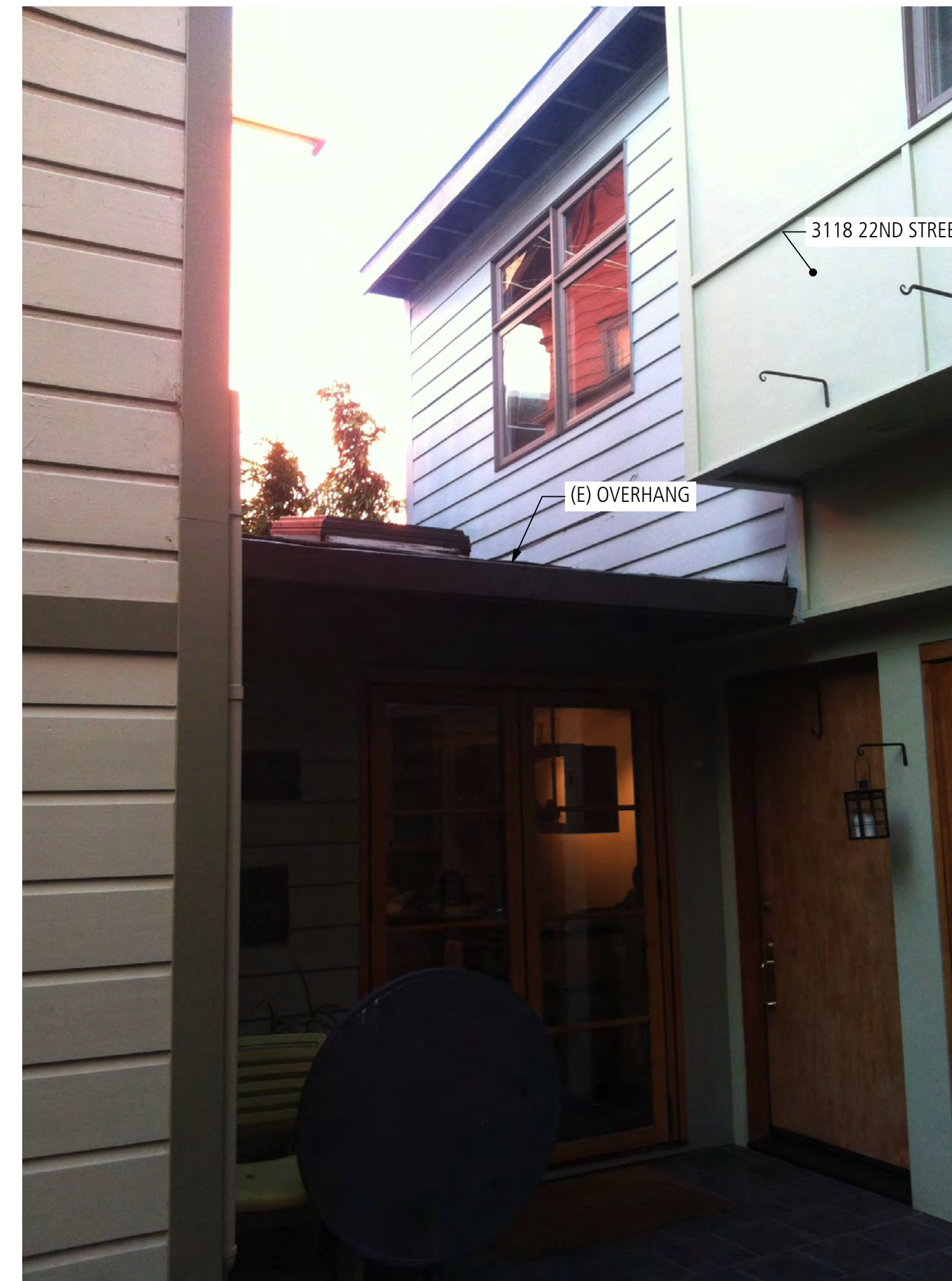
5 A1.01 VIEW 5: EXISTING ROOF OVERHANG @ REAR
