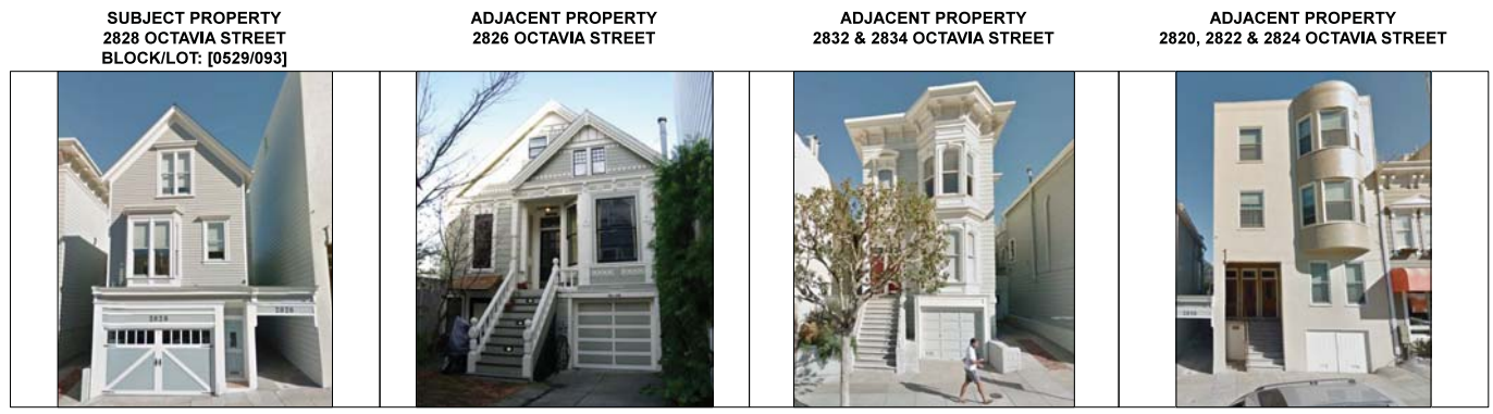
1 BUILDING WEST (FRONT) FACADE
