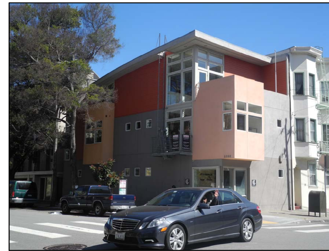
VIEW OF THE BUILDING'S SOUTHWEST CORNER ②
