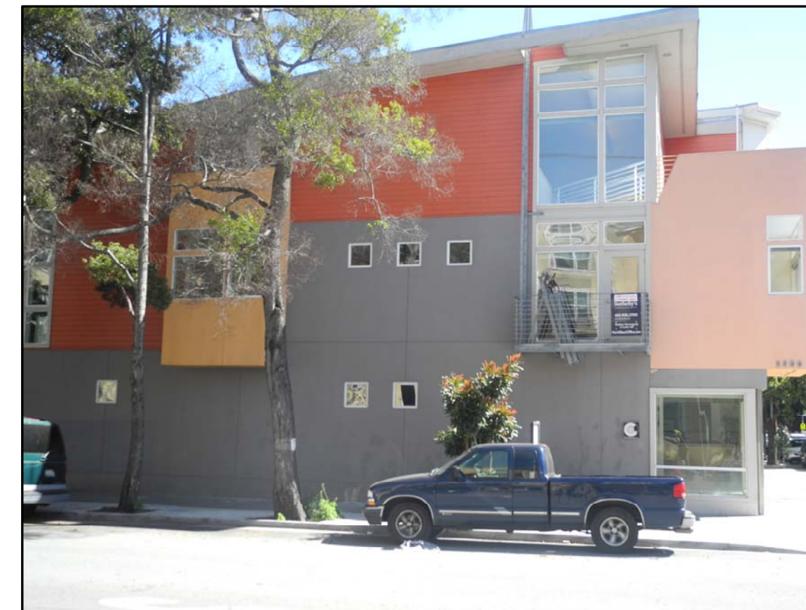
VIEW OF THE BUILDING'S WEST ELEVATION ④
