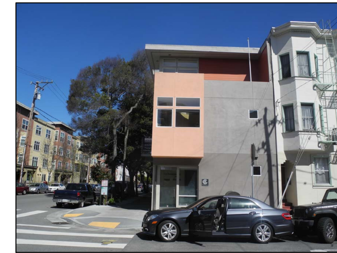
VIEW OF THE BUILDING'S SOUTH ELEVATION ①
