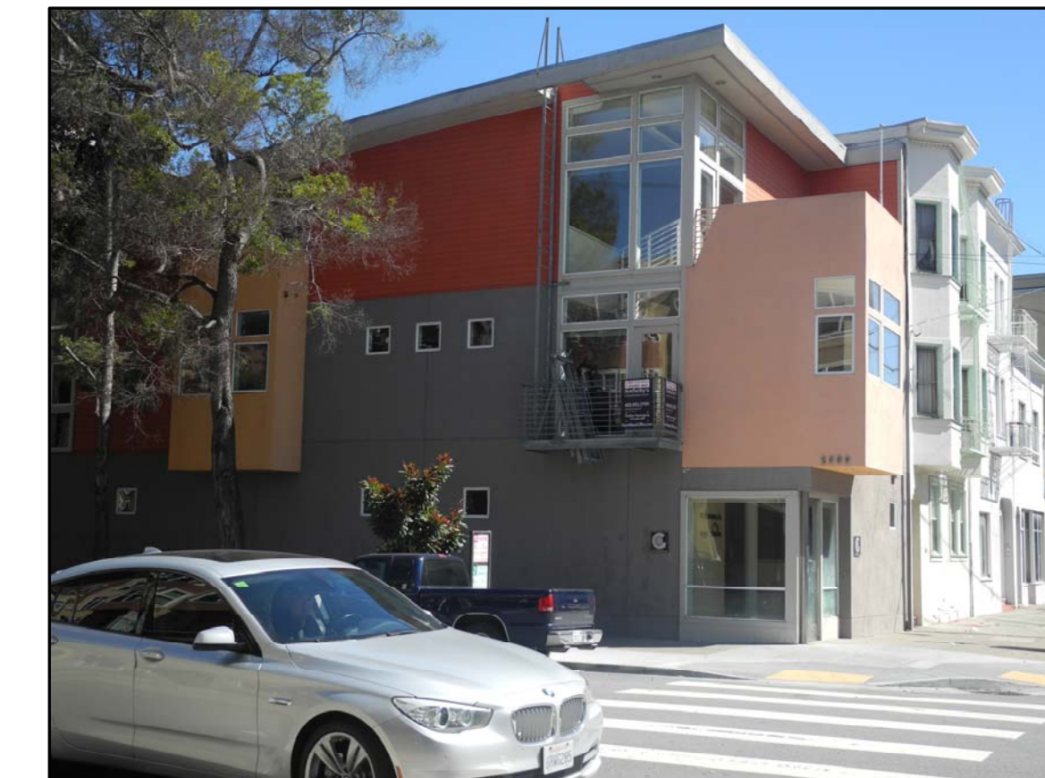
VIEW OF THE BUILDING'S SOUTHWEST CORNER ③
