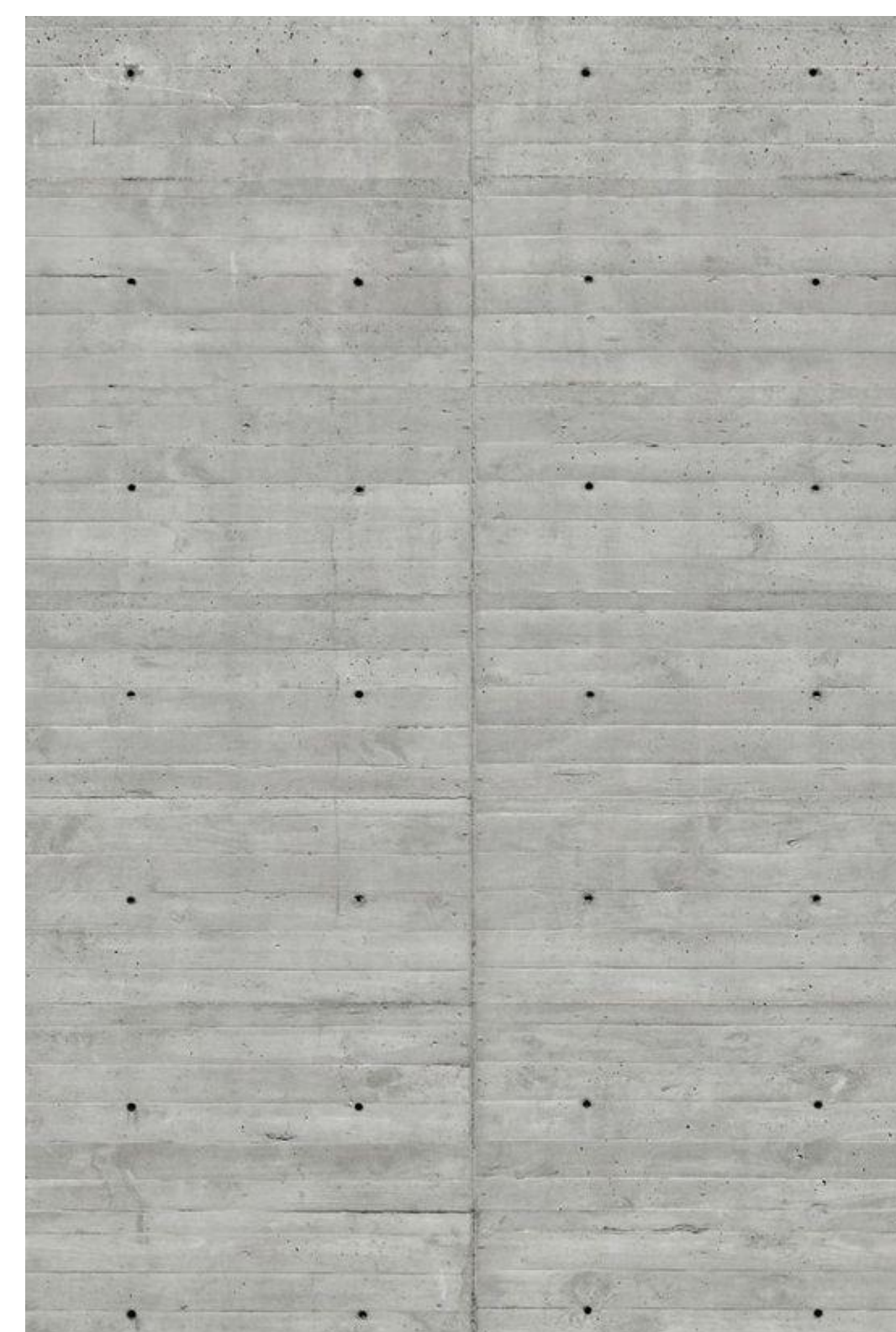
2 CNC 2_BOARD FORMED CONCRETE
