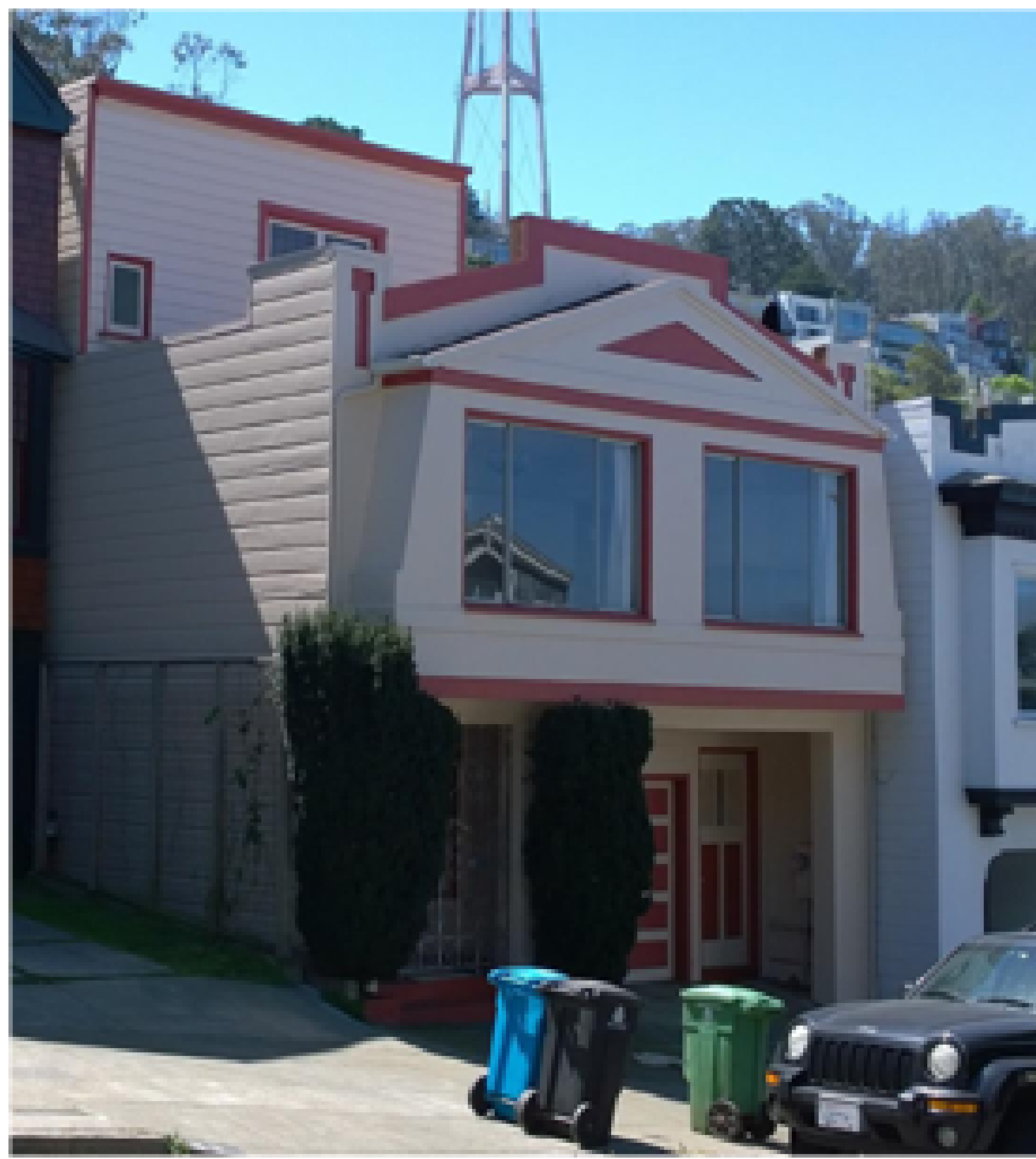
63 CARMEL; FRONT ELEVATION SUBJECT PROPERTY
