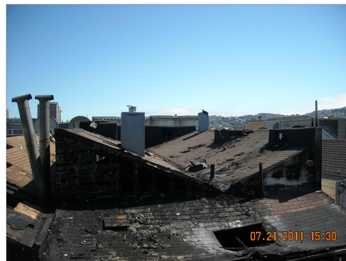
7. ROOF AT REAR OF PROPERTY
