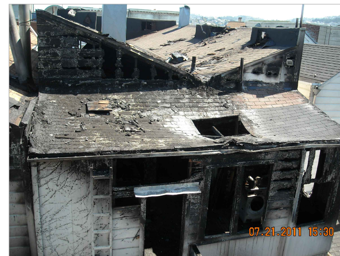
8. ROOF AND SECOND FLOOR AT REAR OF PROPERTY
