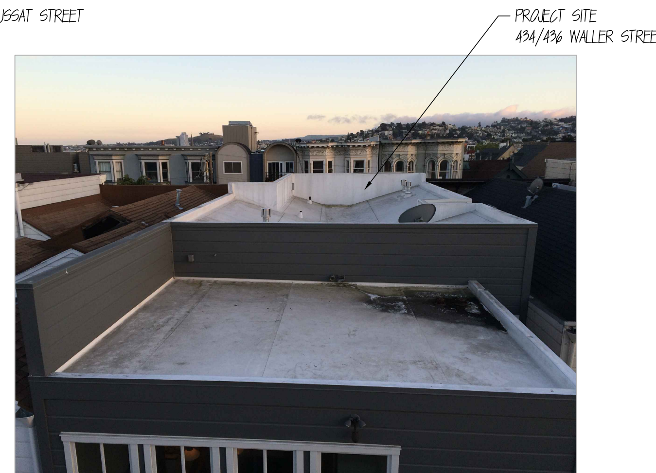
10. PHOTOGRAPH OF ROOF - REFER TO PHOTOGRAPH OF PRIOR ROOF CONDITION 1/A3.0
