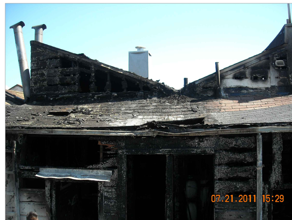
4. ROOF AT REAR OF PROPERTY
