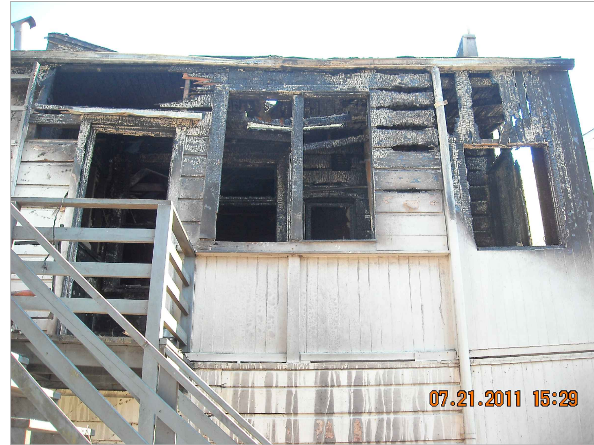
2. BACK OF HOUSE & STAIR ACCESS AT SECOND FLOOR
