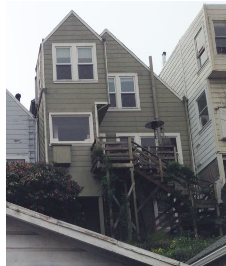
8. ADJACENT PROPERTY - REAR - WEST OF SUBJECT PROPERTY
