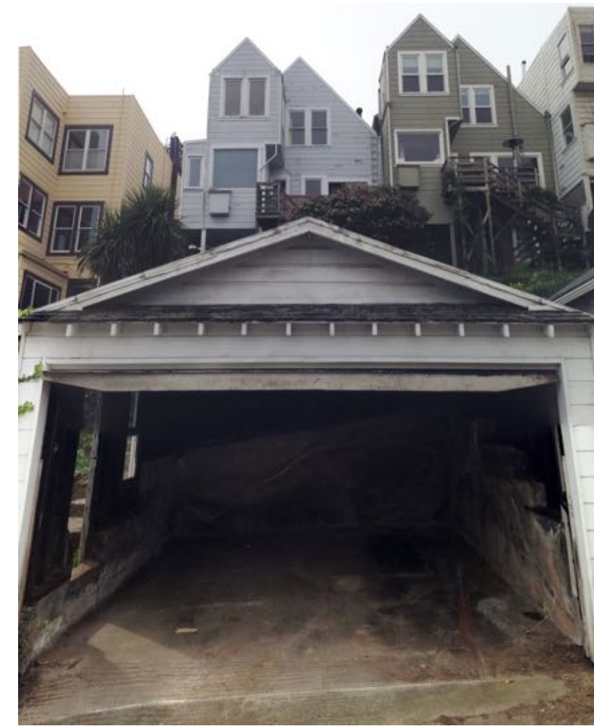
7. SUBJECT PROPERTY - REAR WITH GARAGE
