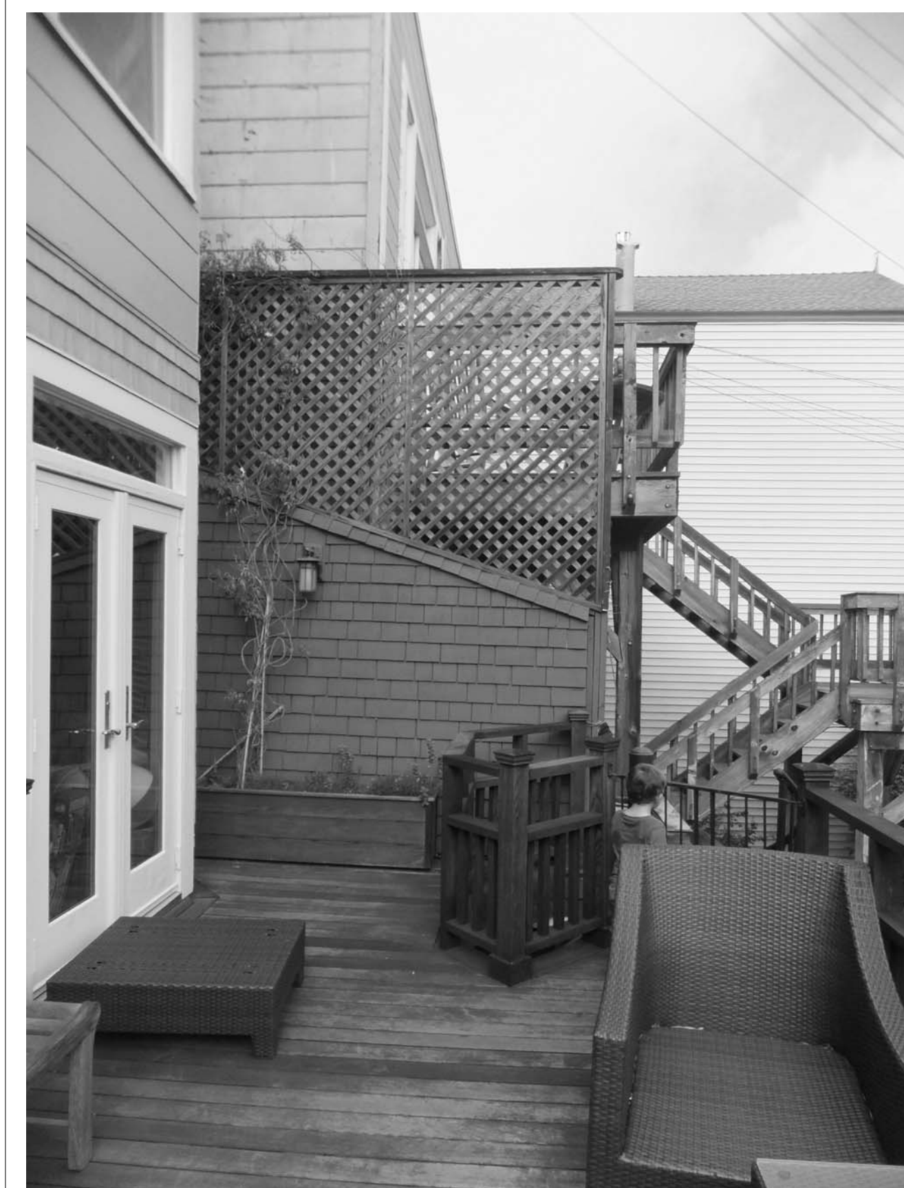
Property Line Wall at Deck (Looking East)
