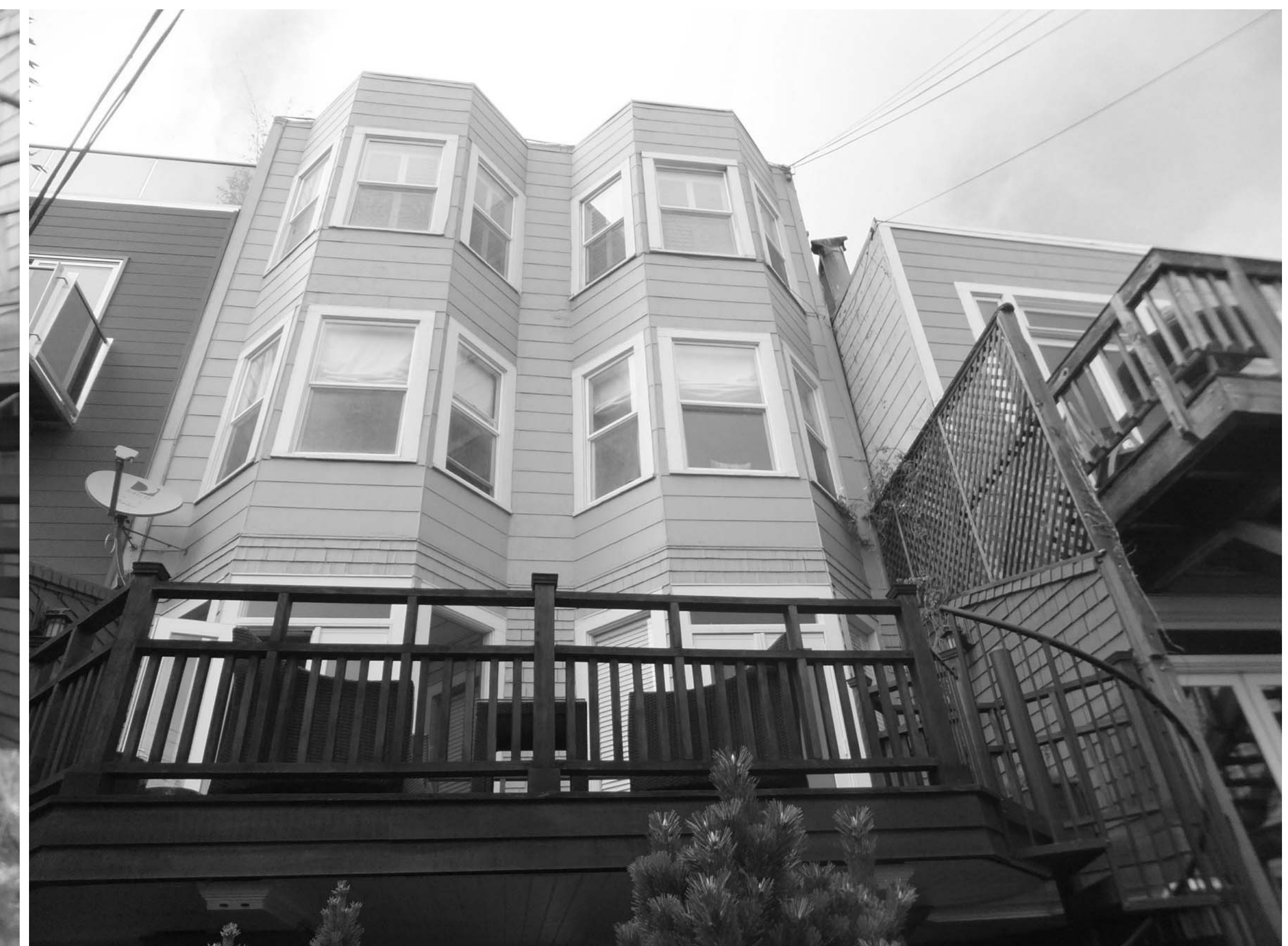
Rear Facade (Deck, Second, Third and Fourth Floors - Looking North)
