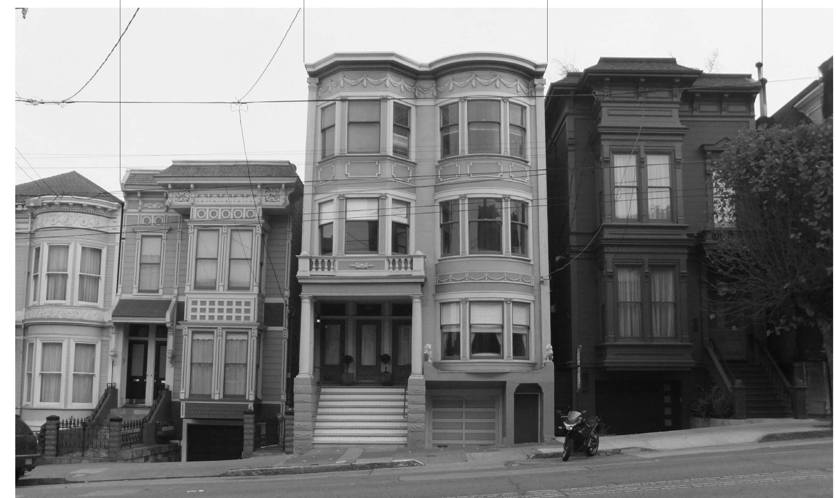
Front Facade (California Street - Looking South)
