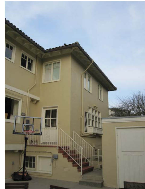
VIEW FROM SOUTH OF SIDE STAIRS
