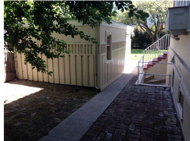
VIEW FROM NORTHEAST OF SIDE STAIRS & GARAGE
