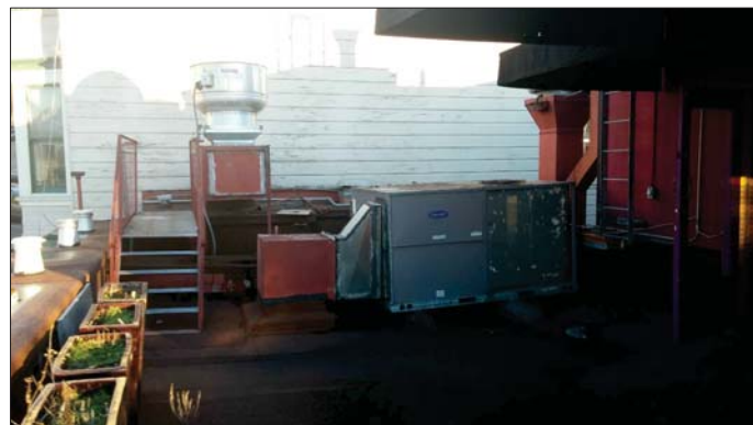
ROOF TOP LEVEL SUBJECT PROPERTY
