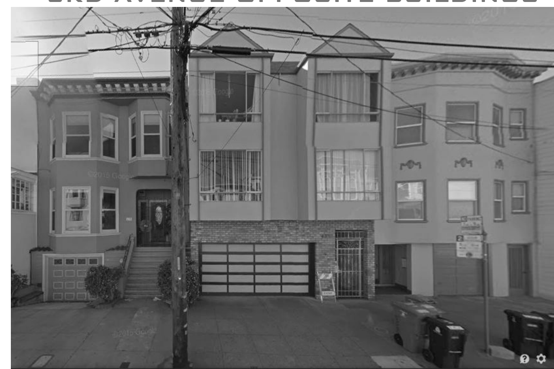
3RD AVENUE OPPOSITE BUILDINGS
