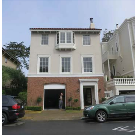
1 PHOTO- SOUTH ELEVATION (FRONT)
