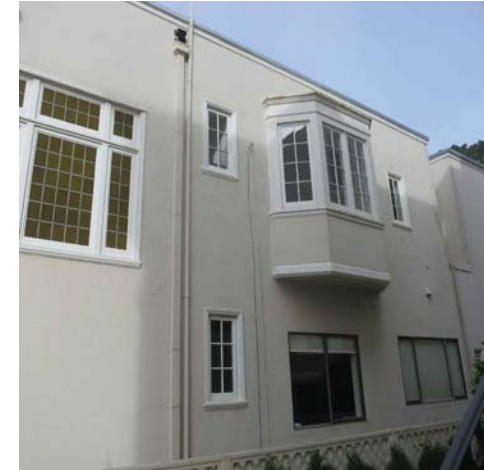
4 PHOTO- EAST ELEVATION (SIDE)
