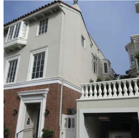
3 PHOTO- EAST ELEVATION (SIDE)
