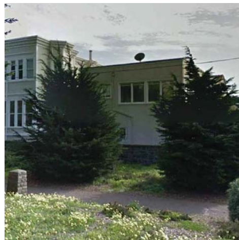
6 PHOTO- NORTH ELEVATION (REAR)
