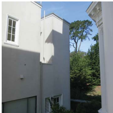
5 PHOTO - EAST ELEVATION (SIDE)
