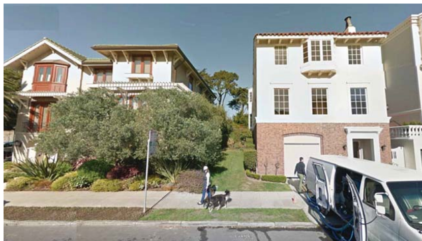
7 SUBJECT PROPERTY & NEIGHBOR TO THE WEST @ 3898 JACKSON
